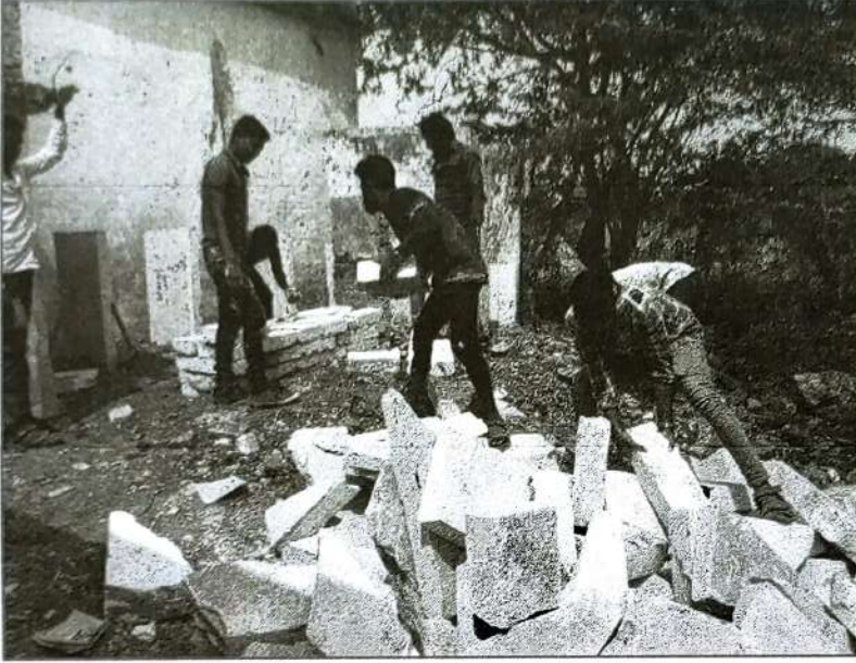
N.S.S Volunteers constructing toilets for students in Govt. School, Tonasanahalli(s)
